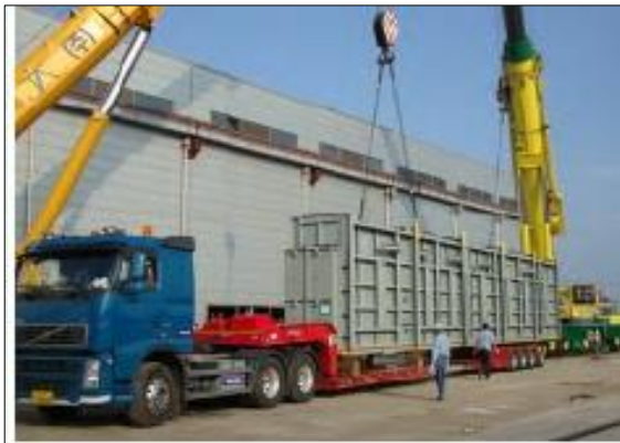
The above photographs show the process of handling the ODC heaters.
